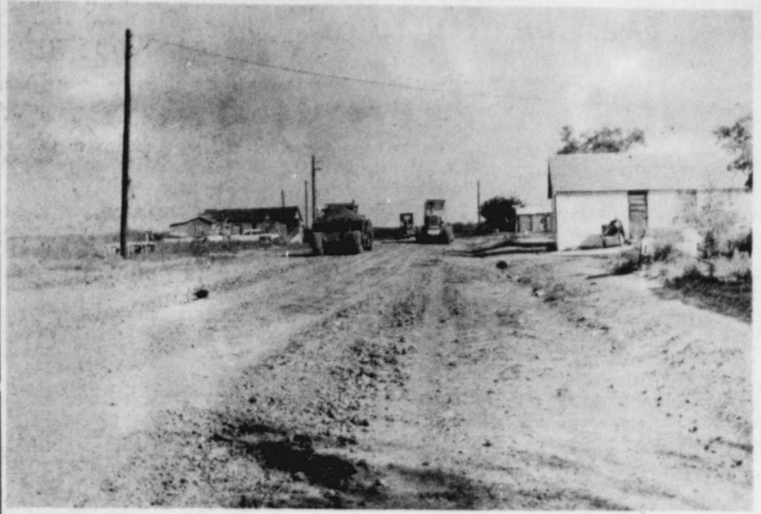
NEW STREETS FOR DELLA PLAINS area of Floydada. Floyd county commissioners began moving caliche onto the Della Plains area streets this week, in a plan to create better streets and drainage for this area of Floydada. (Staff Photo)
