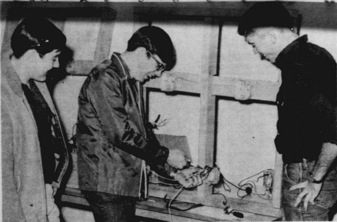
WIRING EXERCISE - Craig Gilly, Kenneth Bloys and Steve Ferguson are pictured above practicing the wiring of a 3-way switch. The FFA members are Ag III students. (Staff Photo)
