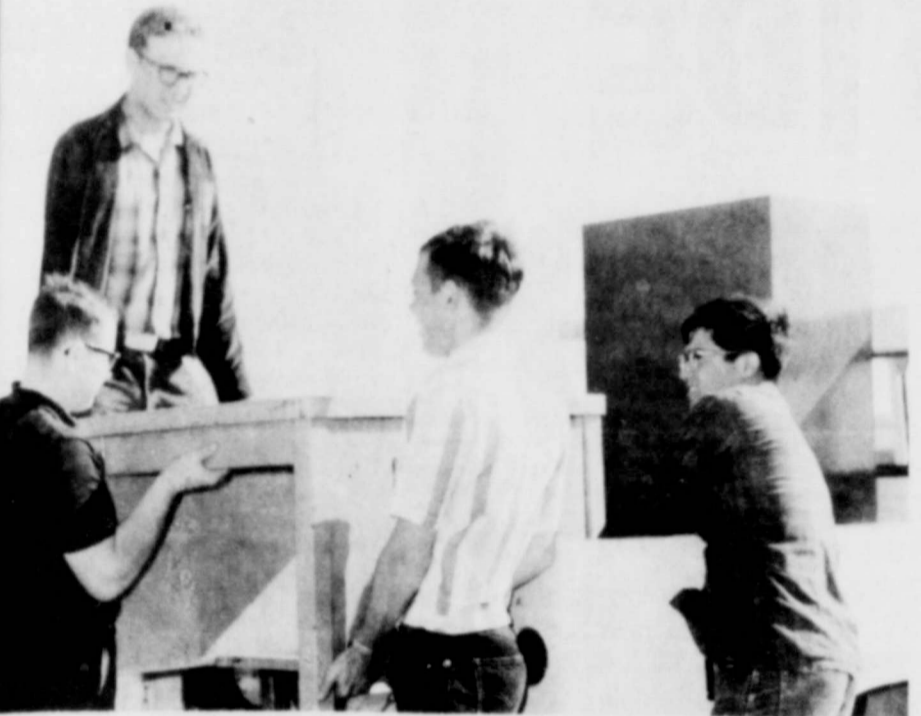
THE BIG BOYS HELPED... high school boys took out of long enough to help unload the heavy furnishings of the new school. (Staff Photo)
