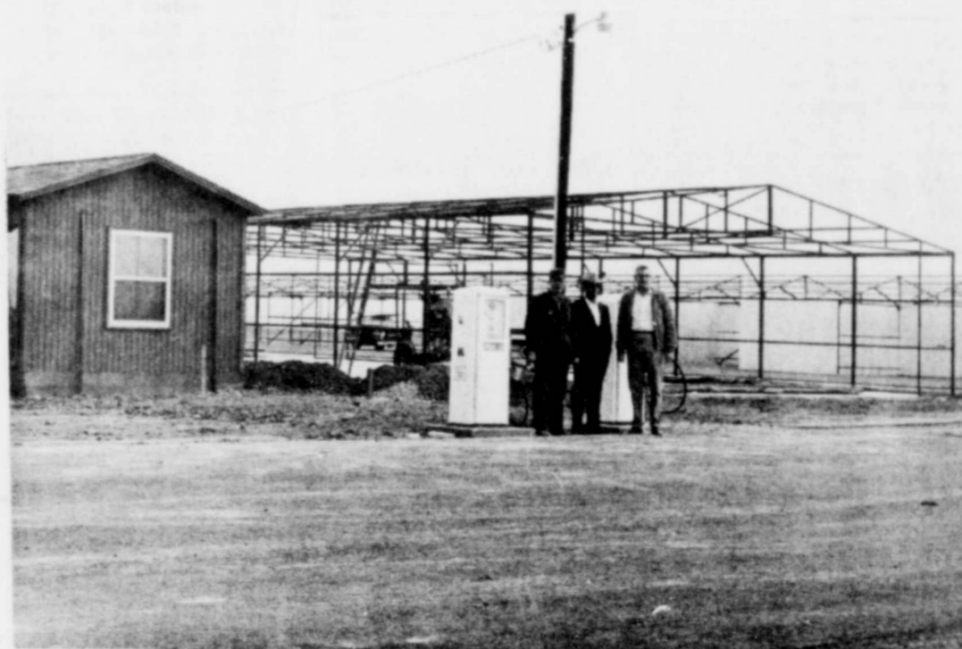
NEW AIRPORT GOING UP. . . MO. STAPLETON, CONTRACTOR
