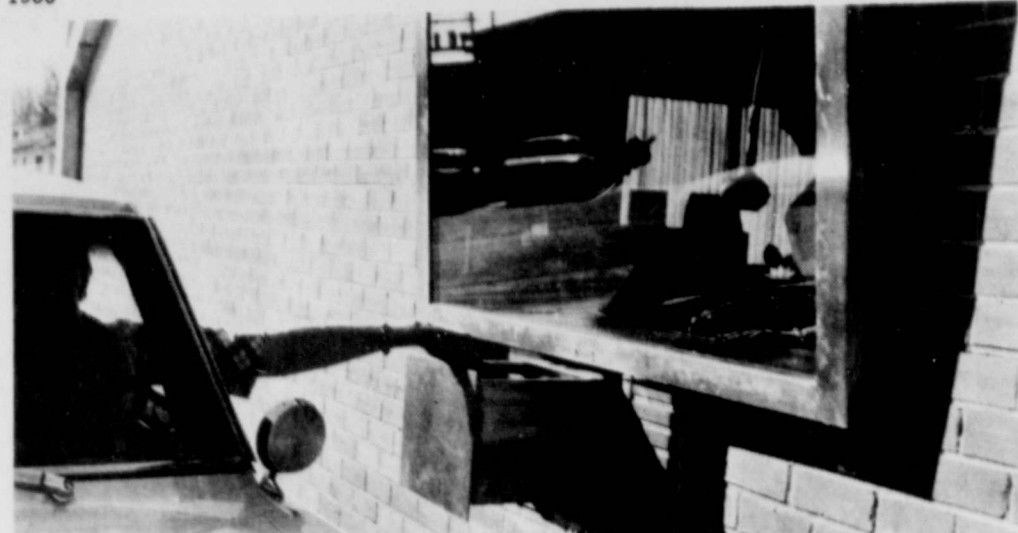
NEW DRIVE IN WINDOW - at Southwestern Public Service in Floydada enables the customer to more conveniently pay bills. (Staff Photo)
