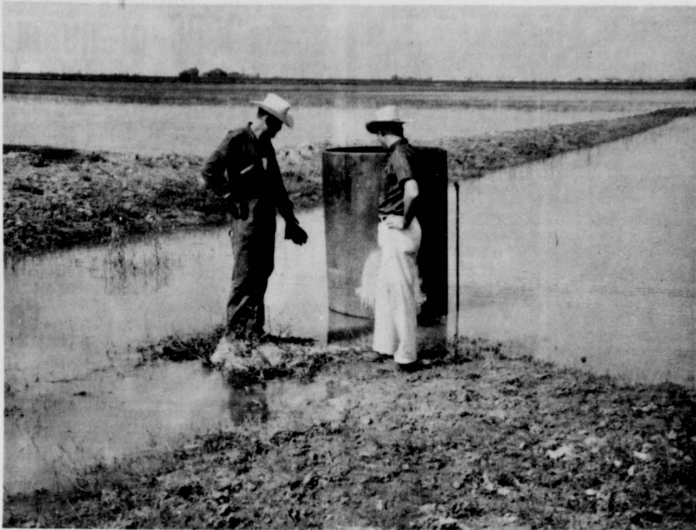
DRAINAGE PIT - Floydada farmer Al Galloway (left) and Douglas Barthosh, soil engineer look at drainage pit in Galloway lake. The water drains from this concrete settlement pit via underground pipe to the irrigation well that is located a short distance to the right.
