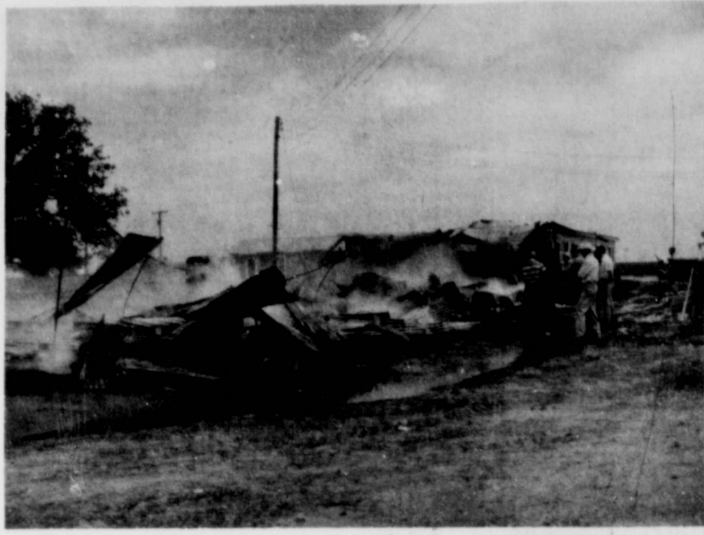
FIRE AT MCCOY - Firemen are shown above attempting to extinguish a blaze at McCoy Gin that broke out Monday morning. Gin employees were attempting to burn weeds from around the barracks when the barracks exploded. It was assumed they had filled with gas from a butane leak. Some tin will be salvaged from the barracks. (Petersburg Post Photo)
