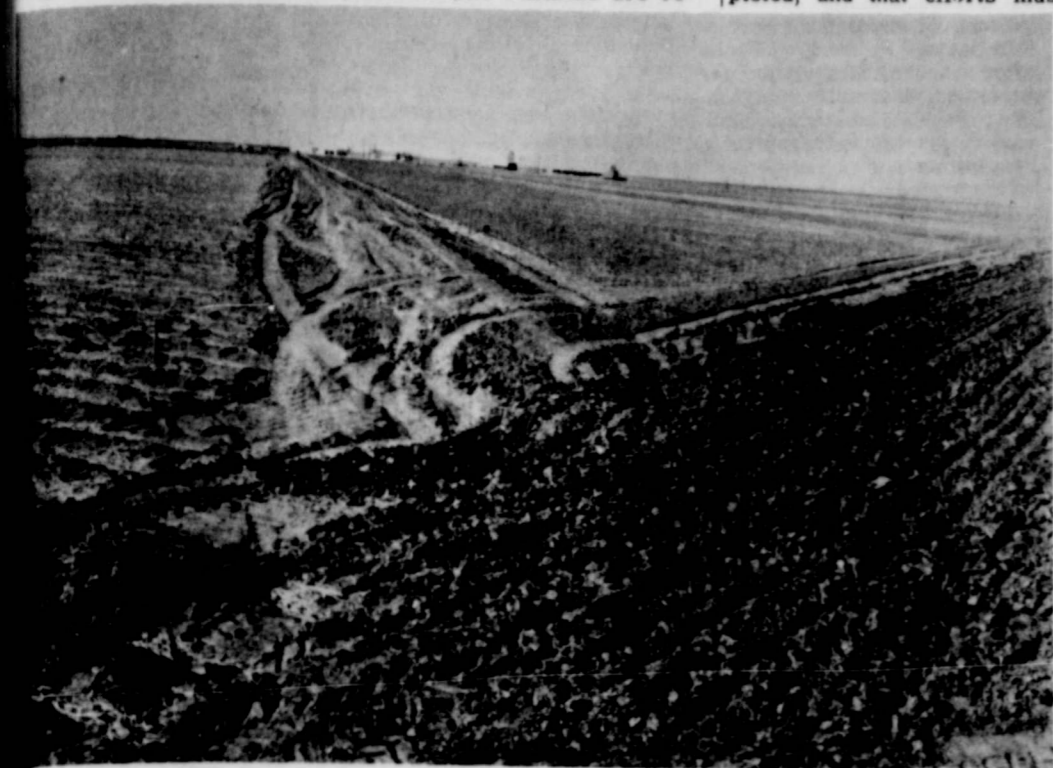
BENCH LEVELED - Pictured above is sloping land which has been bench leveled below a diversion terrace on the C. L. Mooney farm 5 miles north of Lockney. The diversion terrace will protect the bench leveled area. (SCS Photo)
