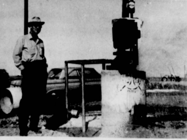
A REAL GUSHER - this lake pump doesn't have the pipe con- nected yet, but Grady Walker flips the switch and it sucks water from an underground pipe that is in the center of the lake on the north side of Floydada. (Staff Photo)
