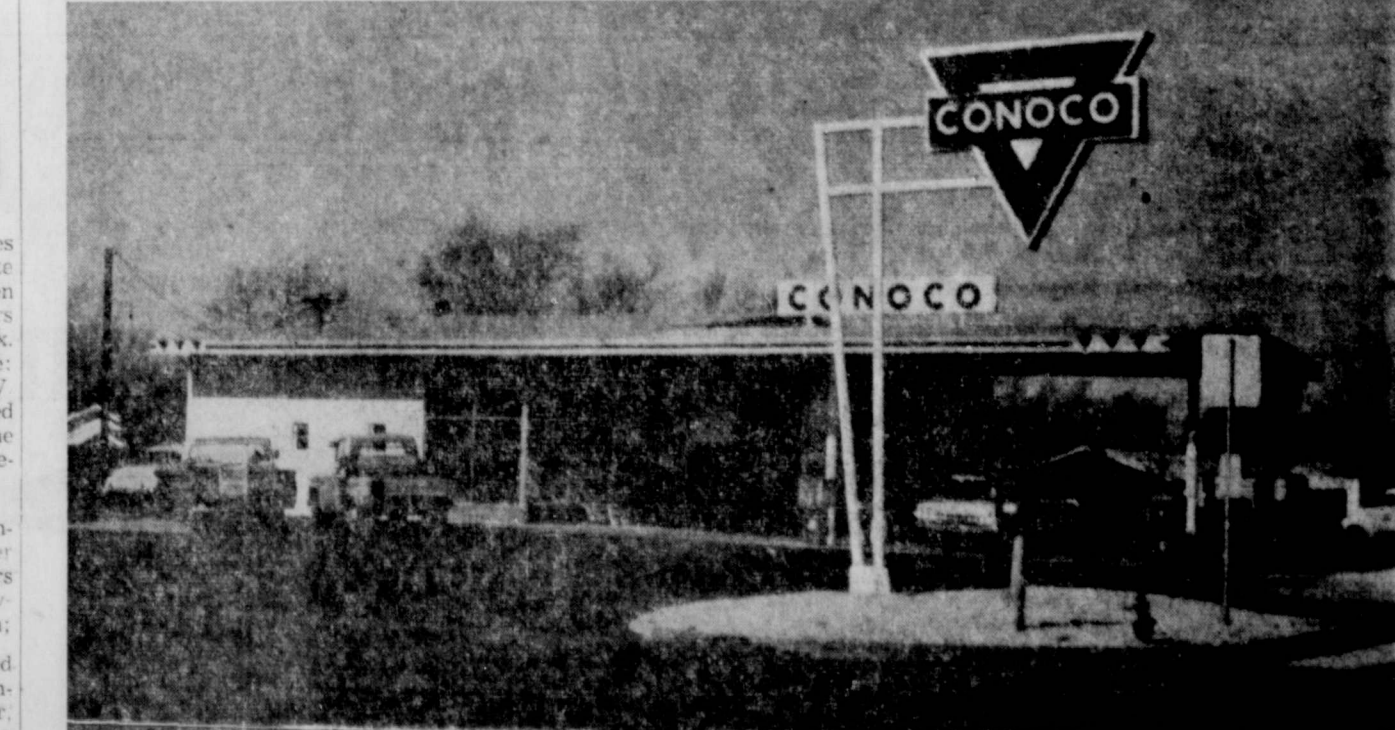
GRAND OPENING SLATED — Shown above is the new McLain's Conoco Station, located at Second and Tennessee streets. The grand opening of the firm has been set for Friday and Saturday of this week at which time a host of prizes will be given away. (Staff Photo)
