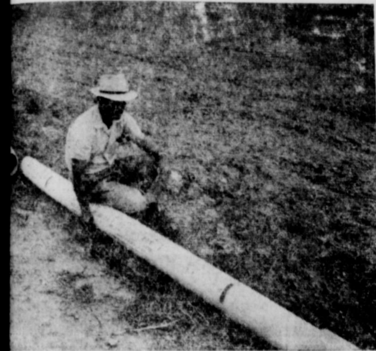
Soil Conservation Technician inspects some asbestos pipe to be installed for a sprinkler system on Leroy Durham farm at Sandhill. This pipe is designed to withstand the pressure required for efficient operation of a sprinkler system.
