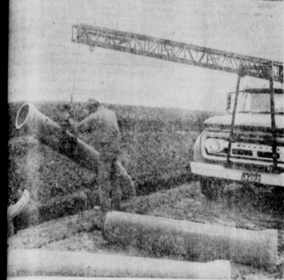
rubber gasket type irrigation pipeline on Joe Dunn farm south of Floyd. The line is being installed to water area adjacent to it that will be established Midland bermuda. Installation of irrigation pipeline is part of Mr. Dunn's overall Great Plains Conservation Program Plan that he developed with assistance from technicians of the Soil Conservation Service.
