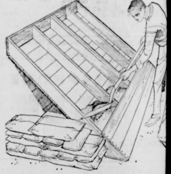
LEAN-TO SHELTER made of lumber would provide protection against fallout in homes with basements, costing less than $75 on a self-built basis, would provide protection as some of the seven other designs in the Defense Department's booklet, "Family Shelter Designs." It combines simplicity of construction, availability of materials, and could be disassembled. Defense offices have the free booklet available now.
