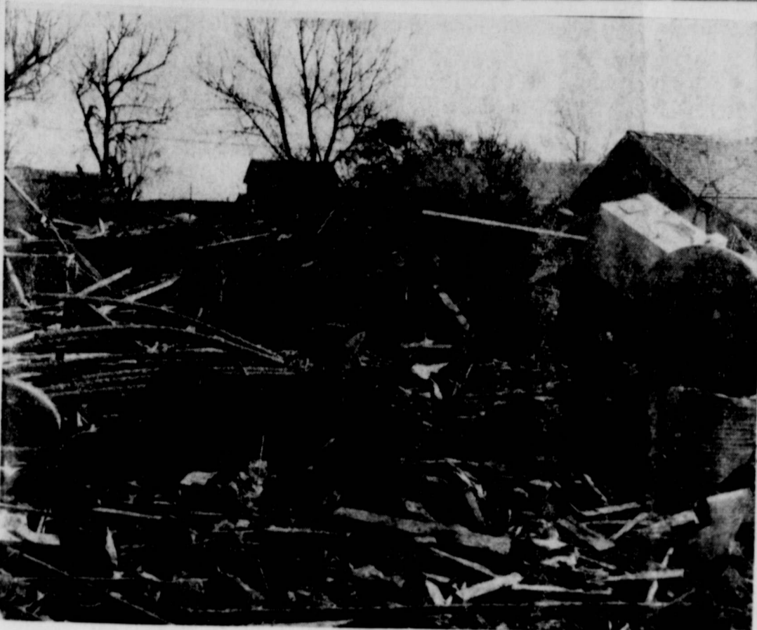
EXPLOSION SCENE. Effects of the terrific early-morning explosion at the Wilks Laundry are shown in this staff photo made by The Hesperian Friday shortly after the accident. The wreckage covers a large number of automatic washers and dryers which the laundry operated. The location is about the middle of the block on Third Street, between Missouri and California Sts., two blocks west of the town square. The building in the background is the Wilks garage at 400 West California. Property east and west of the explosion was damaged more than property north and south. (Staff photo made during a heavy overcast.)
