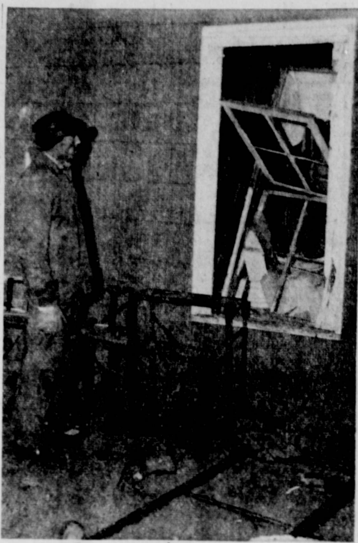
J.W. CANNON views the caved in window in the north end of the Wilks residence, damaged when the Wilks Automatic Laundry, a few feet away, was destroyed by a mighty blast Friday morning at 5 o'clock. (Staff photo)
