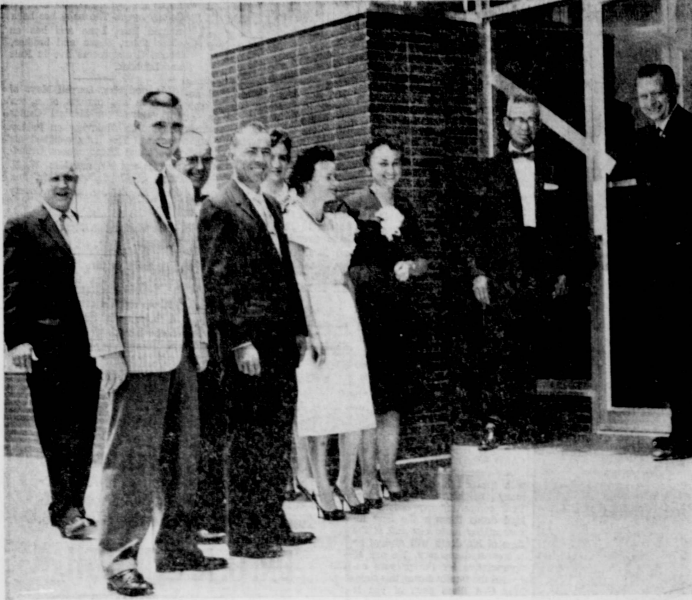
AT THE RIBBON CUTTING — Sunday afternoon there were several visiting officials of Pioneer Natural Gas Company in Floydada to witness the ribbon cutting by Mayor Ross and to help celebrate open house in the company's new building. Pictured here from left to right are R. M. Curry, Lubbock, Pioneer vice president; Wayne Keeter,
