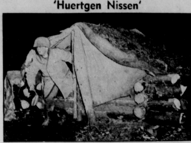
'Huertgen Nissen' It's the Huertgen Forest-style Nissen hut. American soldiers are building them for protection against snow and cold in Germany; chinks of clay, tarpaulin roof, brown paper from cement bags for wall insulation is standard construction. That's Pvt. Theron McCravy of Chester, S. C., who has just heard chow call.
