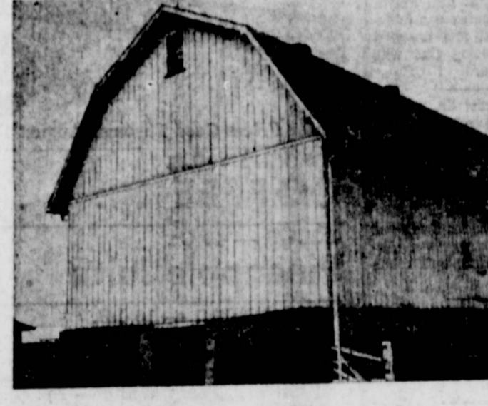
Shelter for livestock for protection against fallout was improved in this barn by using bales of straw as a shield against potentially deadly "post-attack" radiation. Heavy concrete walls, with straw shielding windows, would protect livestock in pens on the barn's lower floor. Barn's upper floor (right) would be covered four bales deep directly above the pens. A shielded room for caretakers, and tractor-powered feed grinder and automatic feeder complete the shelter. (OCDDM Photo)
