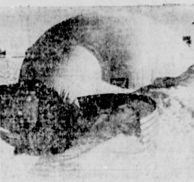
ERSATZ IGLOO—Home in the far north for members of the U.S. Army Polar Research and Development team is this cozy "igloo" made of rubberized canvas and inflated by air. Here a member of the Army team engaged in field research operations clears snow away from the entrance to his air geodesic.
