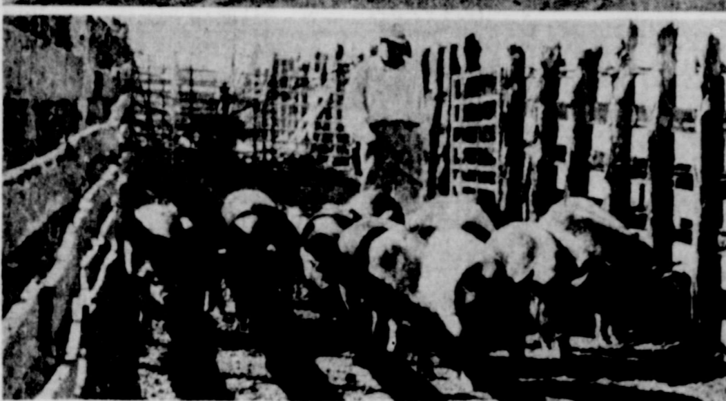
Floydada Live Stock Sales Co. will have their first cattle sale Thursday of next week, Oct. 29, at their new sales arena adjacent to Highway 207 on the northeast outskirts of Floydada. Feverish activity marks the 10-acre plot as completion of pens and interior of the sales barn is under way. The sales building is pictured above, and below an every-day scene as Tom Word, of Brasher & Word, steers a freshly weighed lot of porkers to the holding pens. (Staff photo).
