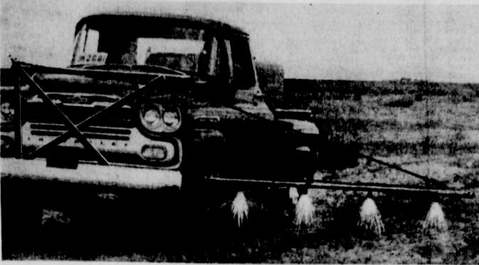
New Spraying Equipment for the control of noxious weeds, capable of covering as much as 10 acres per day, has been put into operation by the county weed control district. Operator hidden in the cab of the pick-up is Bob Hambright. The picture, treated to show off the spraying apparatus, was made by Betty Henry on the Fred Brown farm, north of town.
