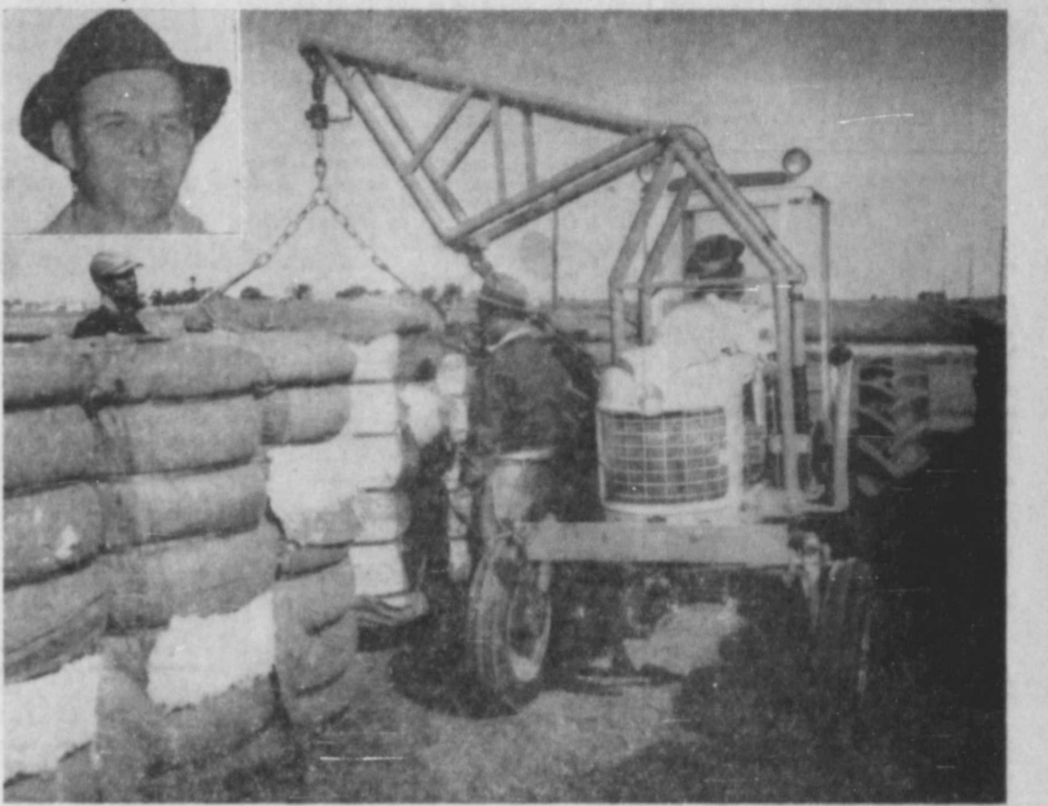
Panhandle Compress and Warehouse Co. received their first cotton in Floydada last Thursday when their water system and fire fighting equipment was readied for operation. Pictured inset upper left is Claude Estes, superintendent of the warehouse plant. Lower shot is that of A. A. Gatman (on tractor) who with a crew is electrically weighing cotton bales on the yard. First days run was 500 bales. The cotton will move into warehouses at it goes into the loan and papers are processed.— Photo by Kenneth Rimmer.
