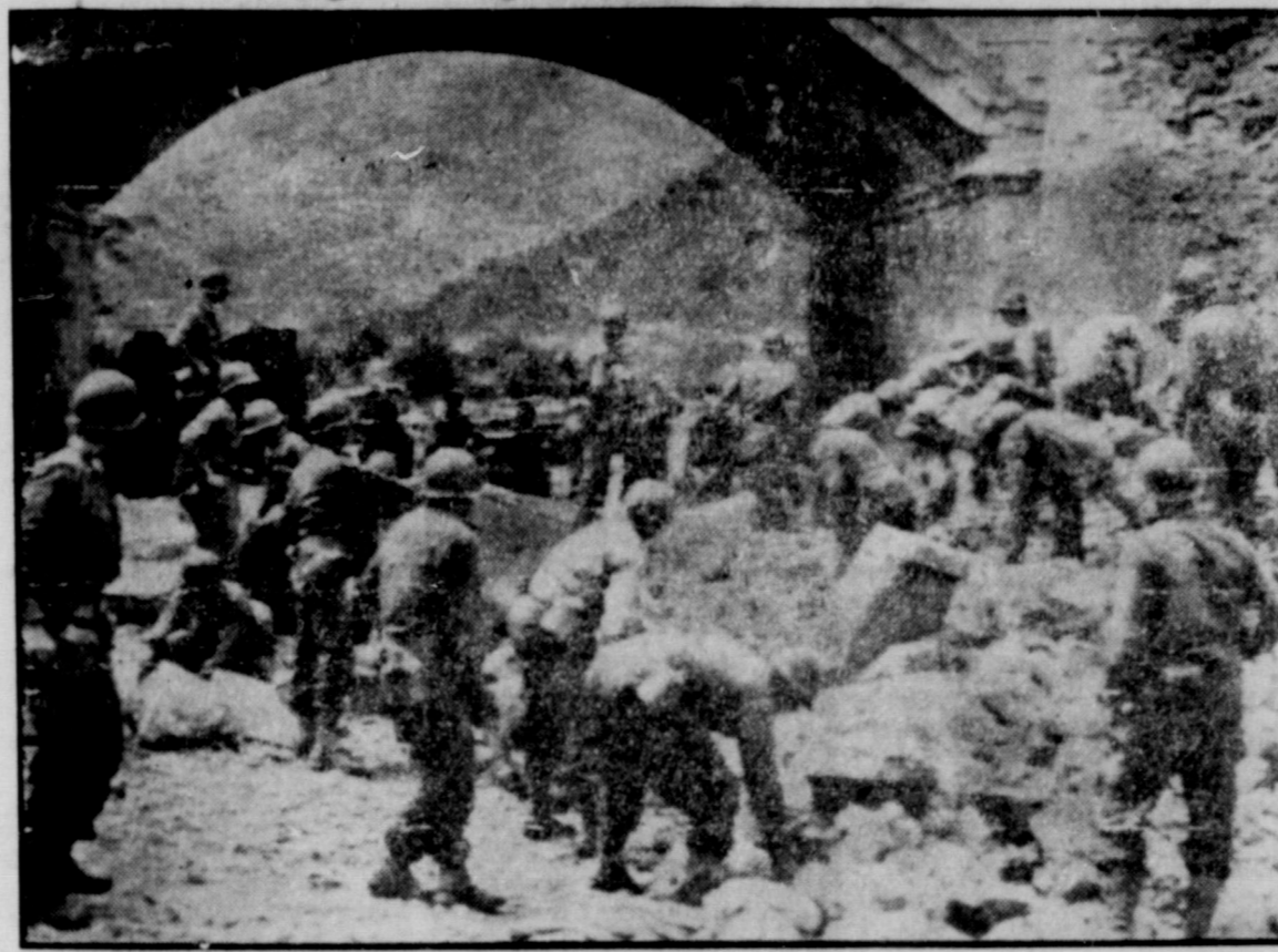
Near Itri, Italy, American engineers clear the blasted Appian Way where it passes beneath a railroad viaduct. This forerunner of the modern super-highway was begun in 312 B. C. by Appius Claudius Caecus the Censor. Succeeding emperors extended it until it terminated at Brundisium (Brindisi) near the Adriatic coast about 244 B. C., furnishing a trade route to the east. Originally it was a two-lane, stone-surfaced highway 15.5 feet wide, 412 miles long. (Army Radio-Telephoto.)
