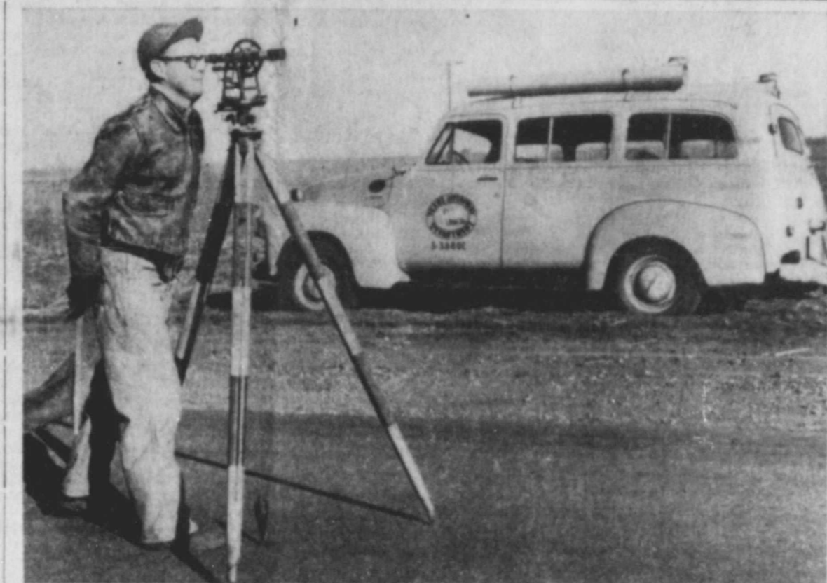
Busy Times are ahead for the field party of Texas Highway Department in Floydada. Here peering into the transit is Glenn White, junior inspector in the resident engineer's office. White, along with fellow crewmembers, is at present running lines on the Lakeview road (FM 651) which is to be redone this year.
