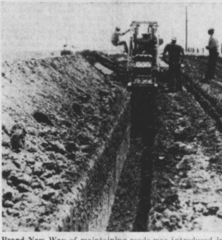
Brand New Way of maintaining roads was introduced in Floyd County last week when ditch diggers were hired to make this 2500-foot cut in an effort to drain water off of the intersection of U. S. Highway 62 and FM 54, six miles south of Floydada. The same tactics are being employed to drain the "Moss Lake" nearer the right of way and was carrying a volume estimated at 3,000 gallons per minute to Blanco Canyon's rim.
