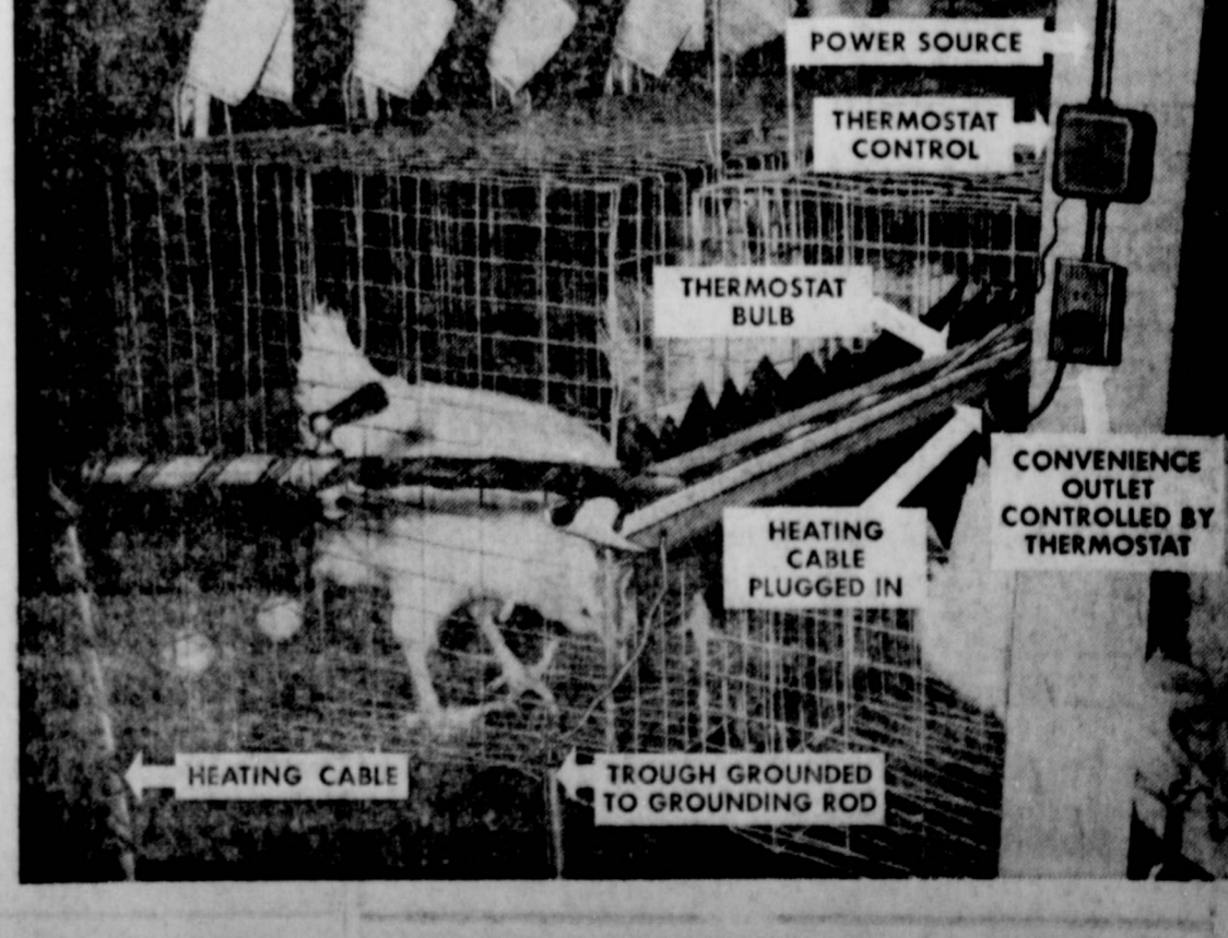
Artist's drawing superimposed over photo shows various parts of water warming installation using electric heating cable. In actual installation, thermostat bulb would be located in center of trough or at opposite end from water source.
