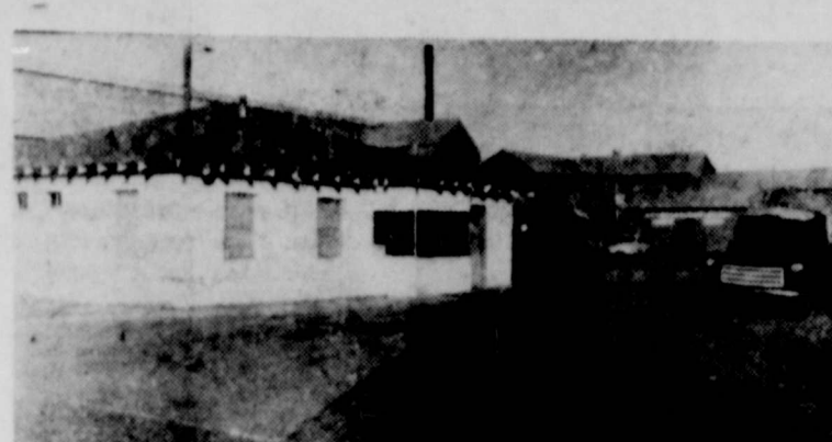
Steadily mounting investment in Floydada gin plants is reflected by this recent $15,000 building program at Farmers Co-Op Gin.
