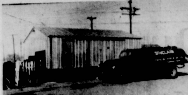
The addition of a Sinclair wholesale agency in Floydada during 1955 led Foote Butane to build this 20 x 30 feet storage unit. Two gasoline storage tanks, not shown, were also added.
