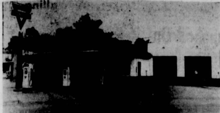
A major modernizing job, costing an estimated $20,000, made over this long established service station at the corner of Fifth and California Streets. Under lease to Continental Oil Company, it is owned by Mrs. R. E. Fry.
