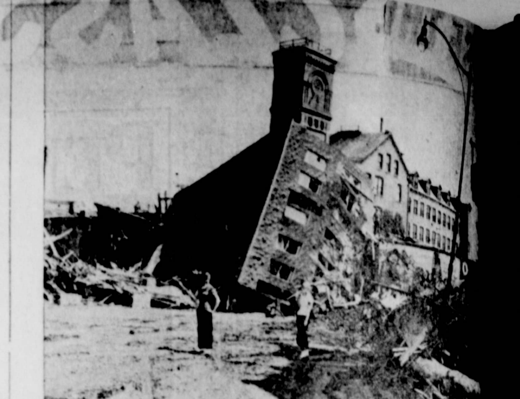
CRUSHED AND BROKEN, this 16-family apartment house in Waterbury, Conn., was left high and dry after the rampaging Naugatuck River receded August 21. This was a sample of the destruction in the flood which, according to the National Flood Insurance Administration, destroyed 1,326 houses and badly damaged many others.
