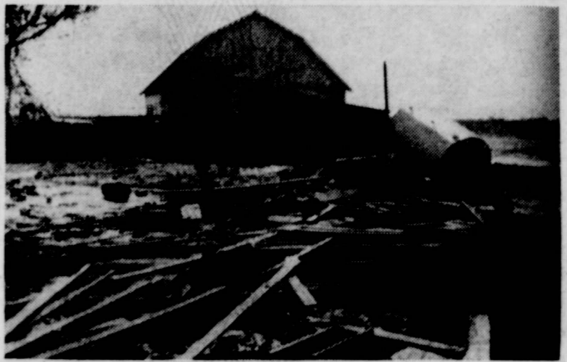
C. M. Perry, 4 miles west of Floydada, lost his hen house, brooder house, tractor house and shop, 96 feet of buildings in Saturday night's storm. Shown left standing but "out of line" is his barn.
