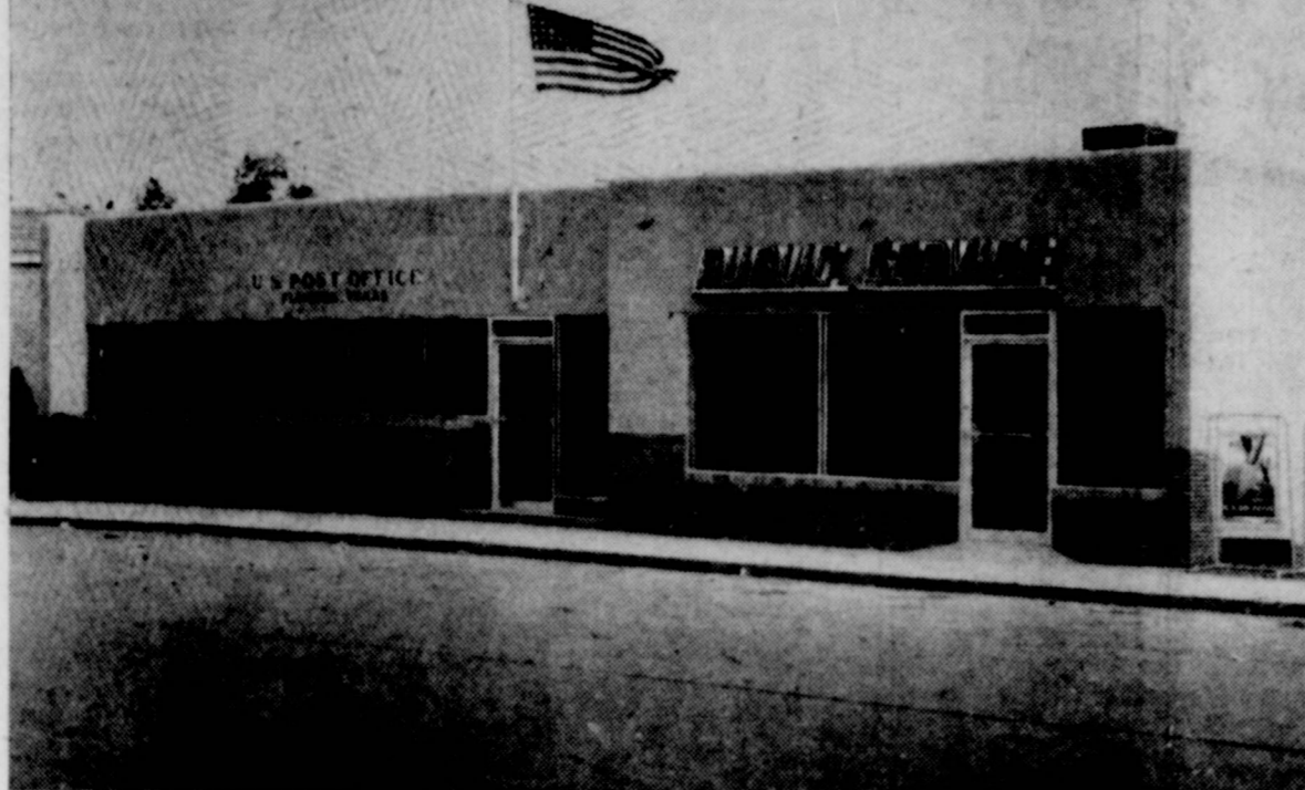
The McDonald Building, housing Floydada post office and Southwestern Public Service Company's office, will be the scene of Friday's open house. Southwestern will make an all-day affair of it. The post office will have "guided tours" in the work shop from 2 to 5 o'clock p. m. The new quarters represent an investment in excess of $30,000 by the builder.
