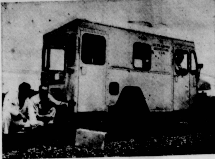
Santa Fe Railway's ultrasonic rail detector car, in operation past two months and believed to be the first of its kind on any American railroad, represents very latest technique in rail maintenance. Hand test machine at rail joint which has reflected faulty indication on car's chronograph recording tape. Pioneered by Santa Fe engineers and equipped for either rail or highway travel, new device picks up more than 95 per cent of all rail defects such as fissures, fractures, bolt hole breaks, separations and other imperfections. Rear picture window provides operators with clear view of tracks as car progresses.
