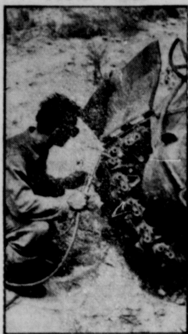
Wearing goggles against the glare of the torch, a 3rd Army maintenance soldier repairs a tank tread on maneuvers in Louisiana. In battle, there often are no garages handy.
