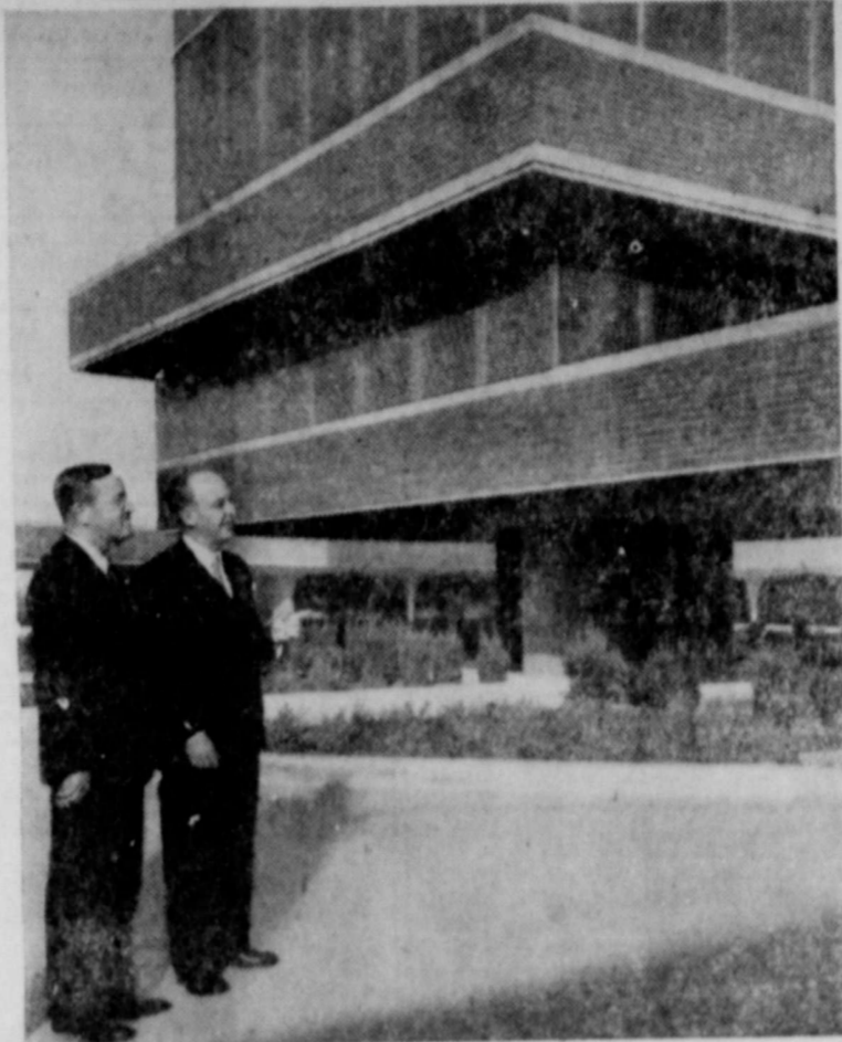
RACINE, WIS.—One of the world's most extraordinary research laboratories was dedicated in Racine, Wis., by S. C. Johnson & Son, Inc., makers of wax products for home, industry and agriculture. Designed by Frank Lloyd Wright, the 153-foot high building has no first floor, no supports directly under the side wall. A central core anchored 54 feet in the ground carries the weight. Twenty-one miles of glass tubing circle the building between bands of brick. The company president, H. F. Johnson, right, is here pointing out the features of the building to Dr. Roger Adams, head of the University of Illinois Chemistry Department, who was principal dedication speaker.
