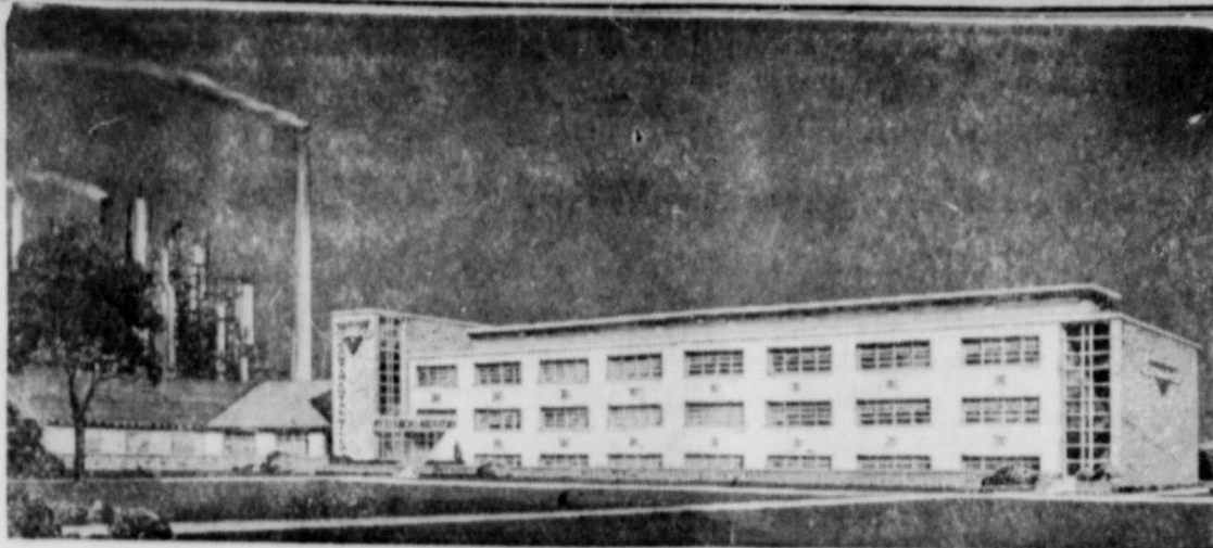
Continental Oil Company has awarded a contract for construction of a $2,250,000 research laboratories building in Ponca City, Okla., that will provide the Company with one of the most advanced development and research programs in the American oil industry, it has been announced by President L. F. McCollum. The new structure, as shown in the architect's sketch above, will be three stories and is expected to be completed in the fall of 1951. Approximately half of the building will be occupied by the Company's central research laboratories, which will include an organic chemical laboratory, a physics research laboratory, for research in electronics, X-ray defraction and mass spectrometry, an analytical laboratory, consisting of both chemical and physical methods units, and a solid laboratory for carrying on fundamental work on greases and allied materials.
