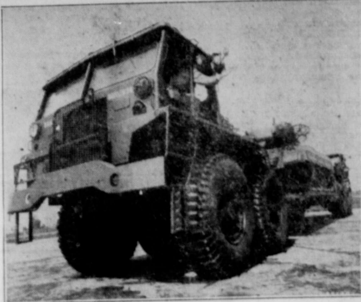
ONE OF THE BIGGEST THINGS IN THE ARMY—This giant T-8 transport, complete with two drivers, one in front and one in the rear, weighs 188,500 pounds when loaded to capacity. Here it transports a medium tank. Its length is 55 feet. The front and rear drivers while on the road speak over the inter-communications radio set. (Official Department of Defense photo).
