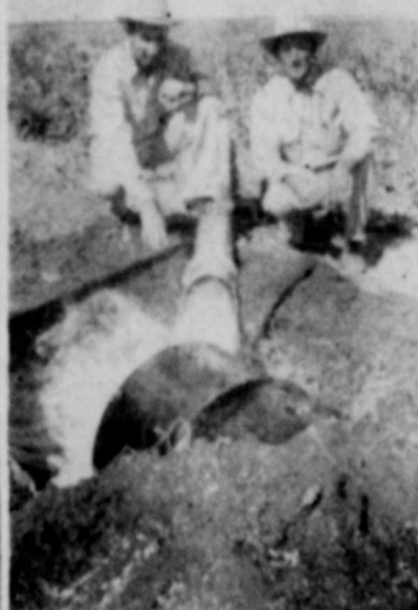
Movable pump and pipe are used to move the water from the lake.
