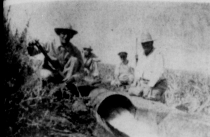
Morckel, left watches water flow through flume which carries the lake water on land that needs the moisture.
