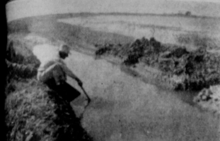
Harry Morckel checks the depth of auxiliary ditch being dug to drain lake on his farm.
