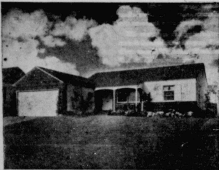
Three-bedroom house, shown above as pictured in the April issue of House Beautiful magazine, is being mass-produced by Henry Kaiser, whose industrial know-how contributed so much to our recent victory. Using partial prefabrication and a standardized floor plan, Kaiser produces dwellings such as these for $8,650. They are located on a 60 x 100 plot. By varying the exteriors, Kaiser has eliminated the dread "rubber-stamp" look of mass-produced dwellings. Housing experts believe the Kaiser technique marks a brand-new development in the housing field, and may solve our national housing shortage.
