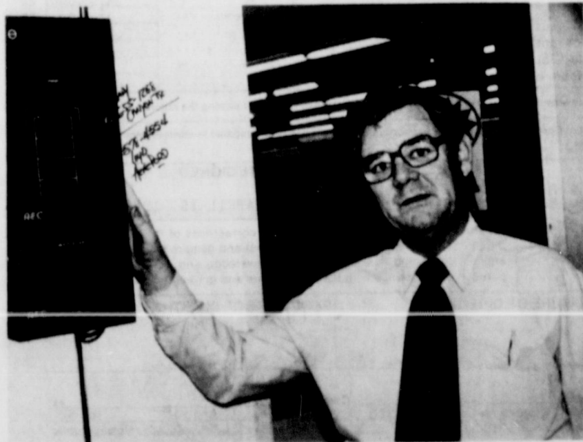
NEW SYSTEM.... Kenneth Moore, owner of Jack and Jill Super Markets in Friona and Hereford, stands beside a new computerized control box he installed in his store, designed to give more economical use of energy, by reducing the "peak" usage periods. A former Friona man, Gary Shackelford, is pioneering High Plains Energy Management Co. of Amarillo, builder of the new system.
