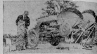
The self-lifting tractor is now a reality. It rises any height, up to four inches, virtually drawing itself up "by its own bootstraps." The lifting operation is accomplished by placing light tubular frame peneath the axles, connecting the rear to the two arms of a Fors Ferguson tractor's hydraulic linkage and lightly touching the "fingentip control" lever which is one feature of the Ferguson System. The antire operation takes less than one minute.
