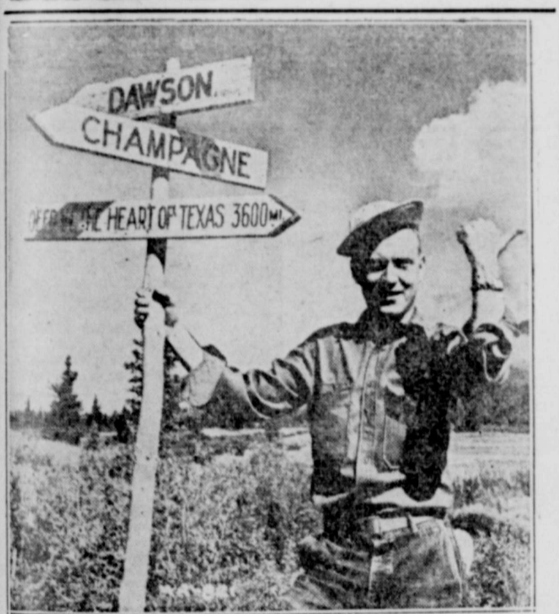
By Bureau of Public Relations, U. S. War Dept., Wash., D. C. NOSTALGIC SIGN POST —Young Army engineers add an extra arrow to a sign post on the route of the Alaska Highway far up in Northern wilderness.
