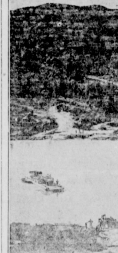
By Bureau of Public Relations, U. S. War Dept., Wash., D. C. ROPE FERRY ON ALCAN HIGHWAY —A typical engineer ferry utilizing the speed of the current to force the boat across by the use of a wire cable stretched from shore to shore.
