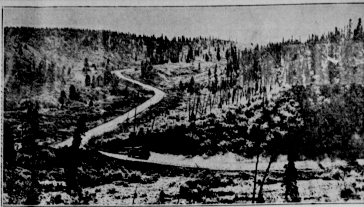
ON THE GREAT ROAD TO ALASKA—A scenic view of a portion of the Alcan Highway where it winds through the wilderness of Yukon Territory. It will be open to traffic early in the winter.
