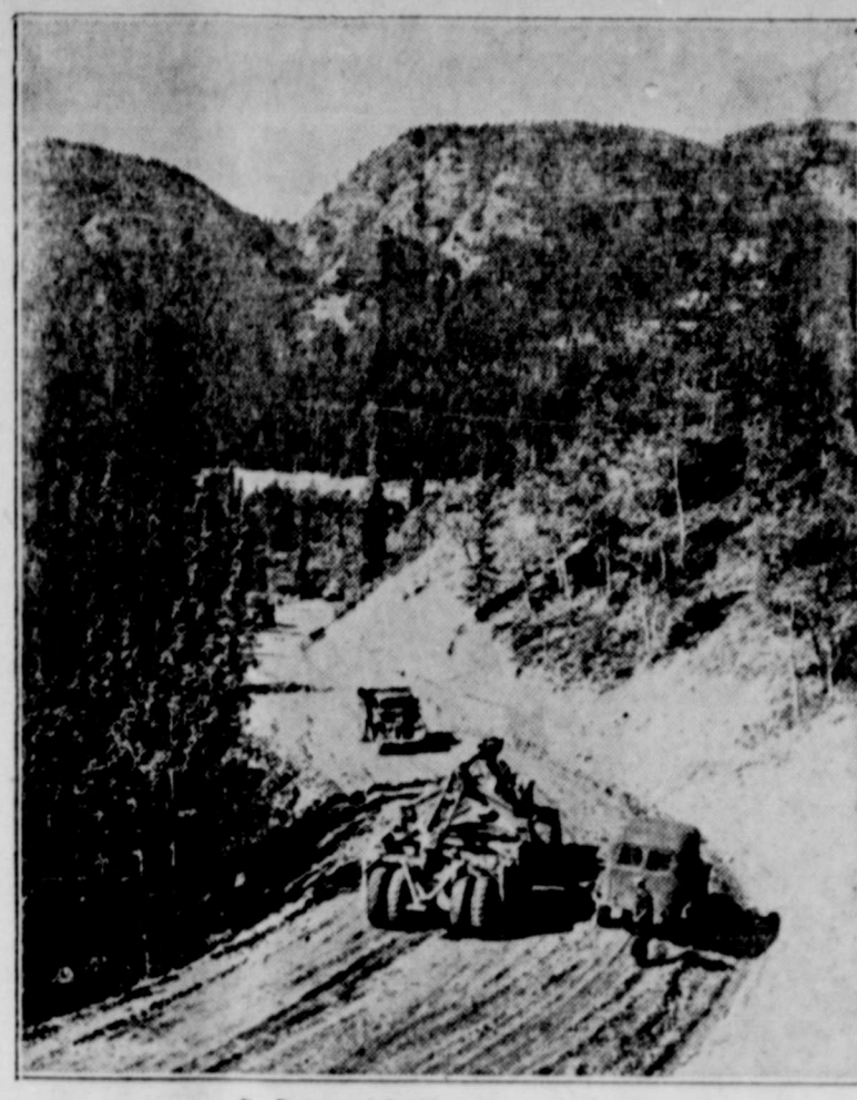
By Bureau of Public Relations, U. S. War Dept., Wash., D. C. ALCAN HIGHWAY UNDER CONSTRUCTION—In the fastnesses of Alaska's mountains the "carry-all" puts the finishing touches on the gravel surface of the great road.
