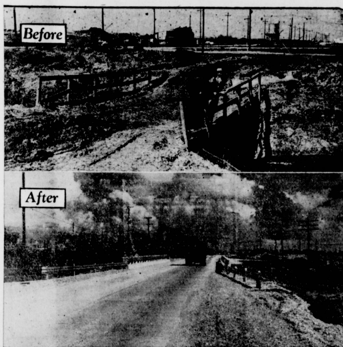
These pictures illustrate how farmers in other sections of Texas are meeting their transportation problems. In the first picture is shown a muddy, virtually impassable road, which in six months was transformed into a high speed, durable highway. Costly? Yes, but it is paying for itself many times over.
