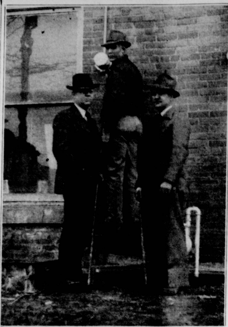
Mayor Glad Snodgrass (left) and city engineer J. L. Puckett (right) look on as L. D. Britton, city lineman, connects the first meter for the new Floydada Municipal Power and Light Plant early in January.
