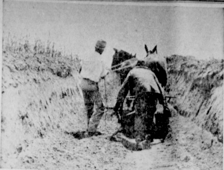
Trench Silo. —Good pictures of trench silos have been hard to make. This one shows August Hegar, 4-H club boy of Hockley, digging a 140-ton silo that he later filled with grain sorghum. He bought steers and fattened them for the market with the silage as roughage.
