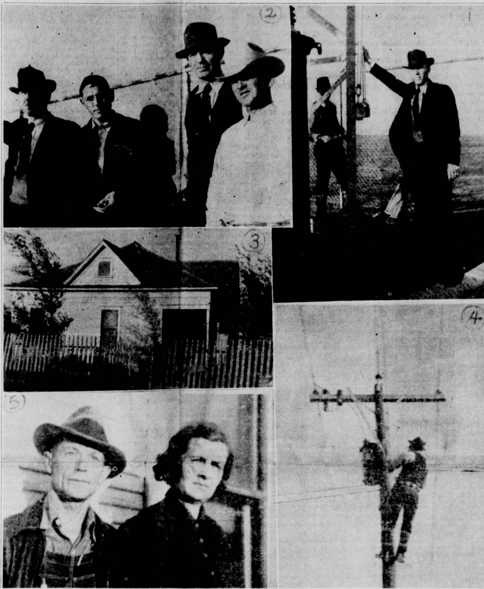
Photos by Bill Hams L. W. Chapman, rural electric superintendent, throws main switch making 175 miles of line "hot" for Floyd and Hale counties. (2) Appearing left to right are L. W. Chapman, A. Chatham-Strode, project engineer; Dona Covington, co-op secretary and bookkeeper; L. D. Britton, linesman, and G. L. Snodgrass, member of the co-op board of directors. (3) Home of Mr. and Mrs. T. B. Rambeau, first farm home to receive rural electricity. (4) L. D. Britton throws fuse switch giving Rambeau home power. (5) Mr. and Mrs. T. B. Rambeau, first users of power from the line.
