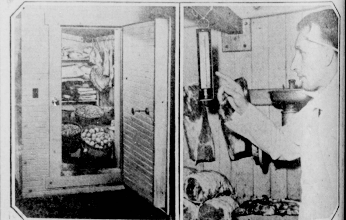
A neatly packed community refrigerator is the Kensington, Ga., unit, shown at left above, filled with a variety of agricultural products and meats. The butcher, right, cuts meat before storage and keeps check on the temperature to assure that the products will keep well.
