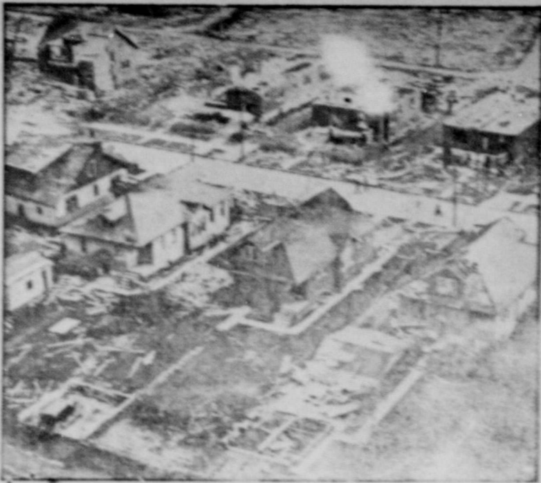
Belleville, Tex., a town of 28,000, received the brunt of the devastating tornado which swept up the Mississippi Valley, as the above photo indicates. Nine in the Illinois town were killed, and 60 buildings were wrecked.
