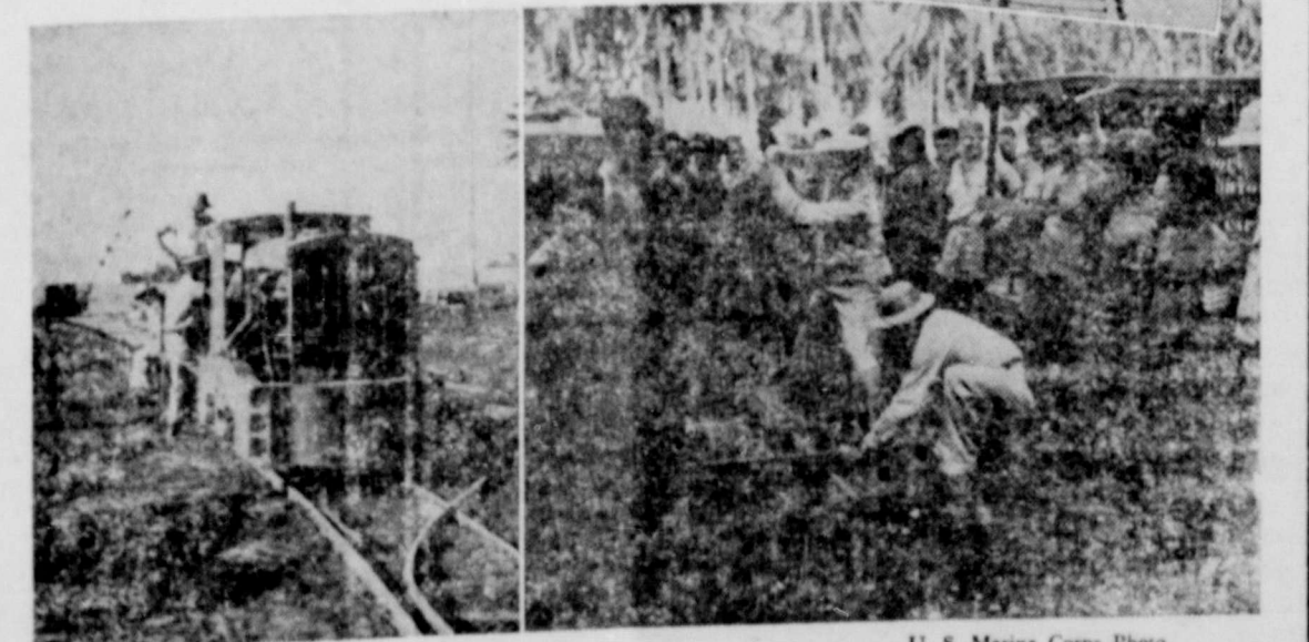
Seabees, members of a Naval Construction Battalion, completed the Guadalcanal Division of the "G. B. & T." (Guadalcanal, Bougainville & Tokyo) Railroad in three days. Photos show one of the line's gas-powered engines, a spur nearing completion, the division's first train and the "last spike" ceremony.
