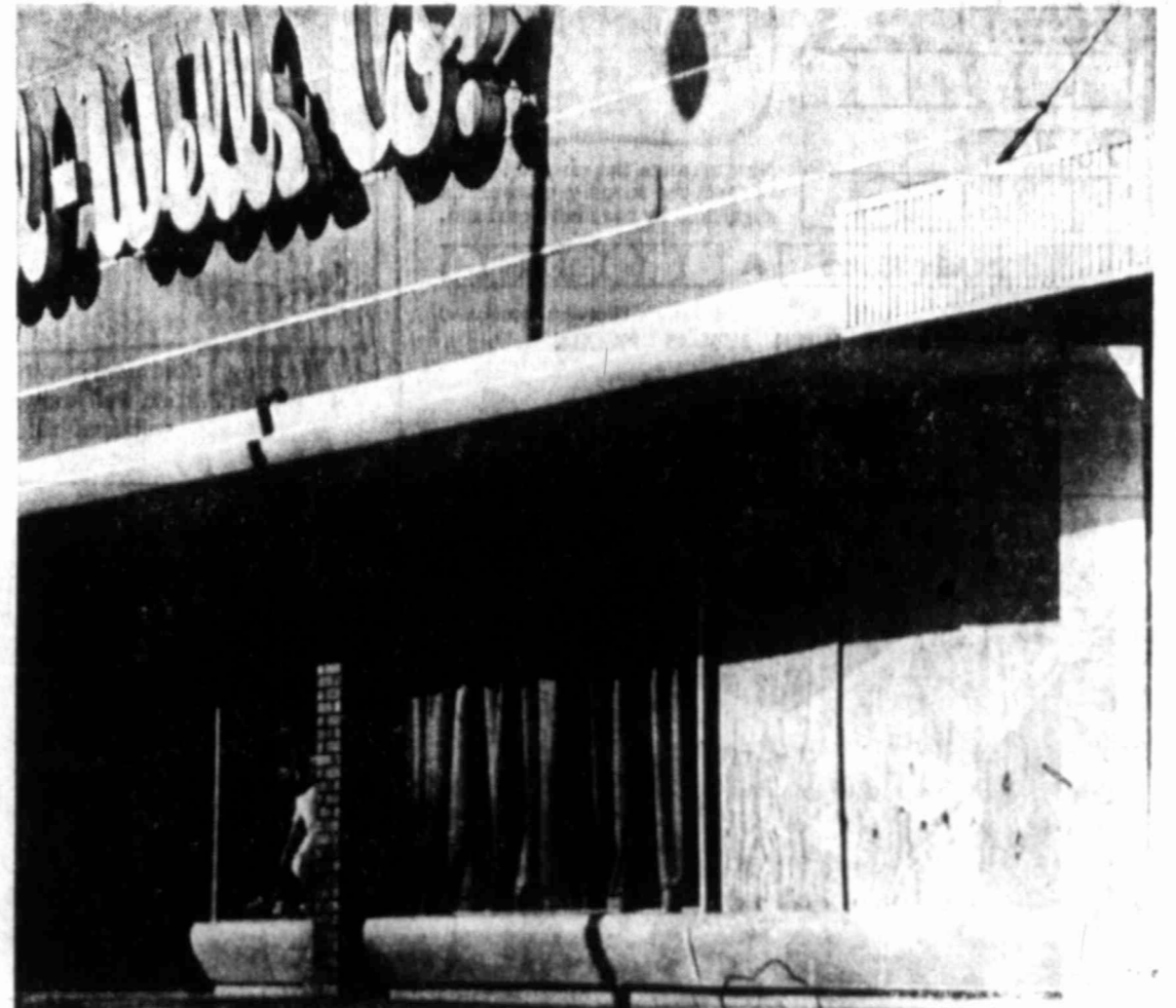
DOWNTOWN DEPARTMENT STORE TAKES A BEATING — Tuesday's high winds battered in downtown Big Spring long enough to blow out several plate glass windows, including the Hemphill-Weils store pictured here. That particular area may have escaped major damage, although complete reports are still coming in.
