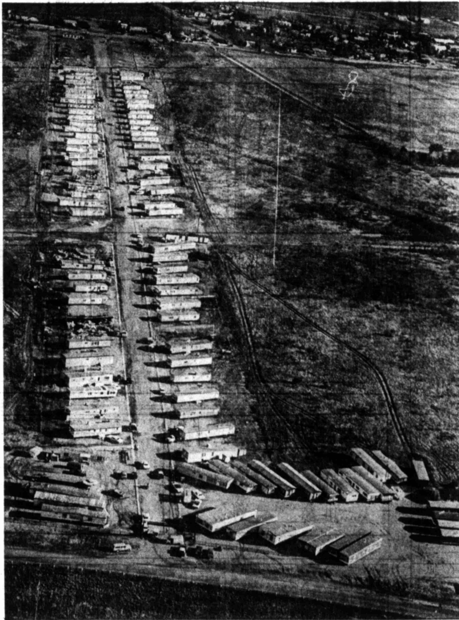
HIT AND MISS ANTICS SHOWN — Not all of the mobile homes at Chaparral Trailer Park were damaged, as this area shot revealed. Some of the structures were torn apart,
