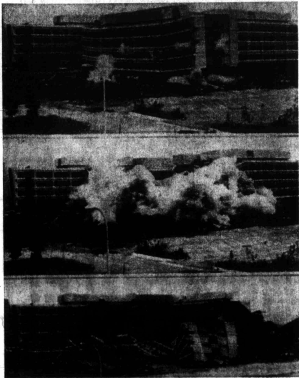
FINAL CHAPTER OF CALIFORNIA'S BIG QUAKE—The walls came tumbling down at Olive View Hospital in the Sylmar section of Los Angeles Thursday as half of the $34 million structure—damaged irreparably in the earthquake of 1971—was demolished by dynamite. Useable equipment had been removed. Three persons were killed in the building during the quake. Demolition will be done in sections.
