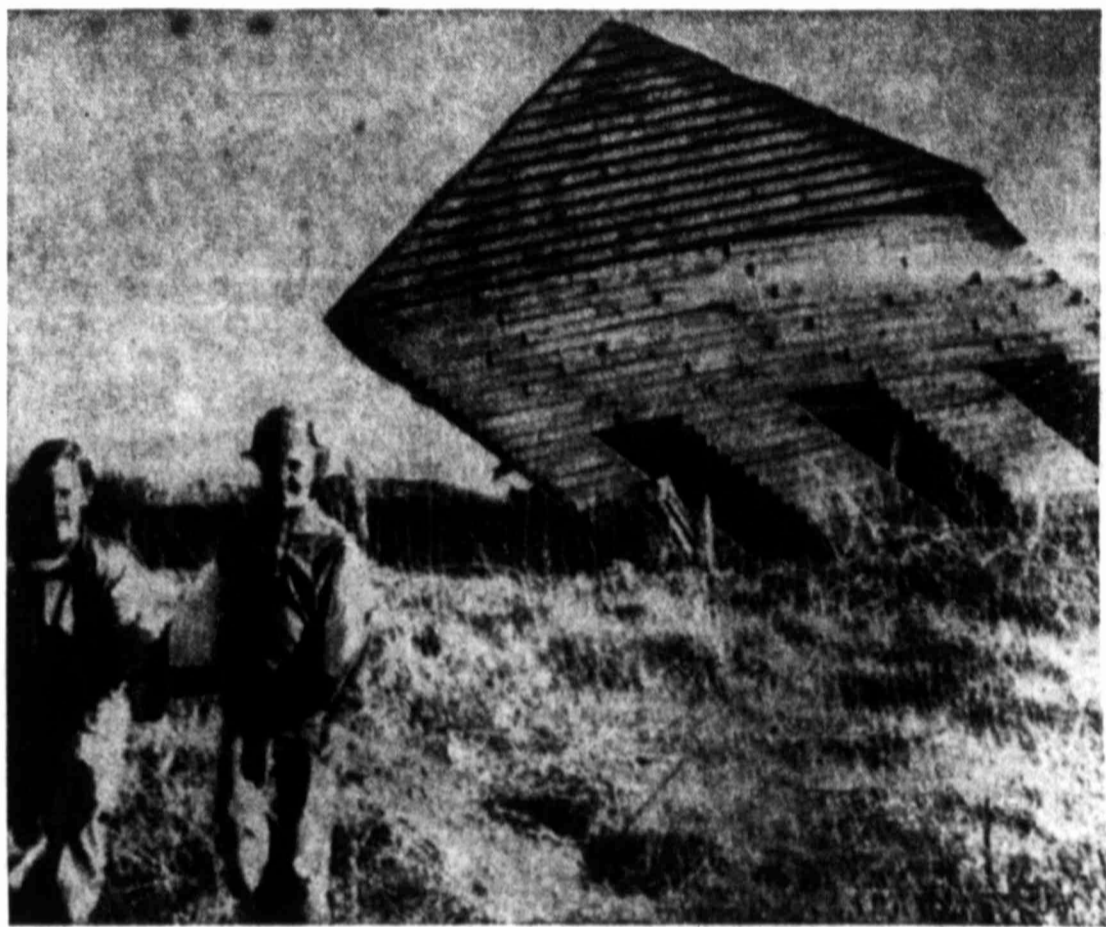
DEFIES GRAVITY — It may not match the Leaning Tower of Pisa as an architectural wonder, but this corn crib near Preston, Minn., has been defying the law of gravity for years. No one seems to know what holds the crib up since there are no supports to keep it from toppling to the ground. Child in the foreground is Debbie Sikkink, who lives on a nearby farm.
