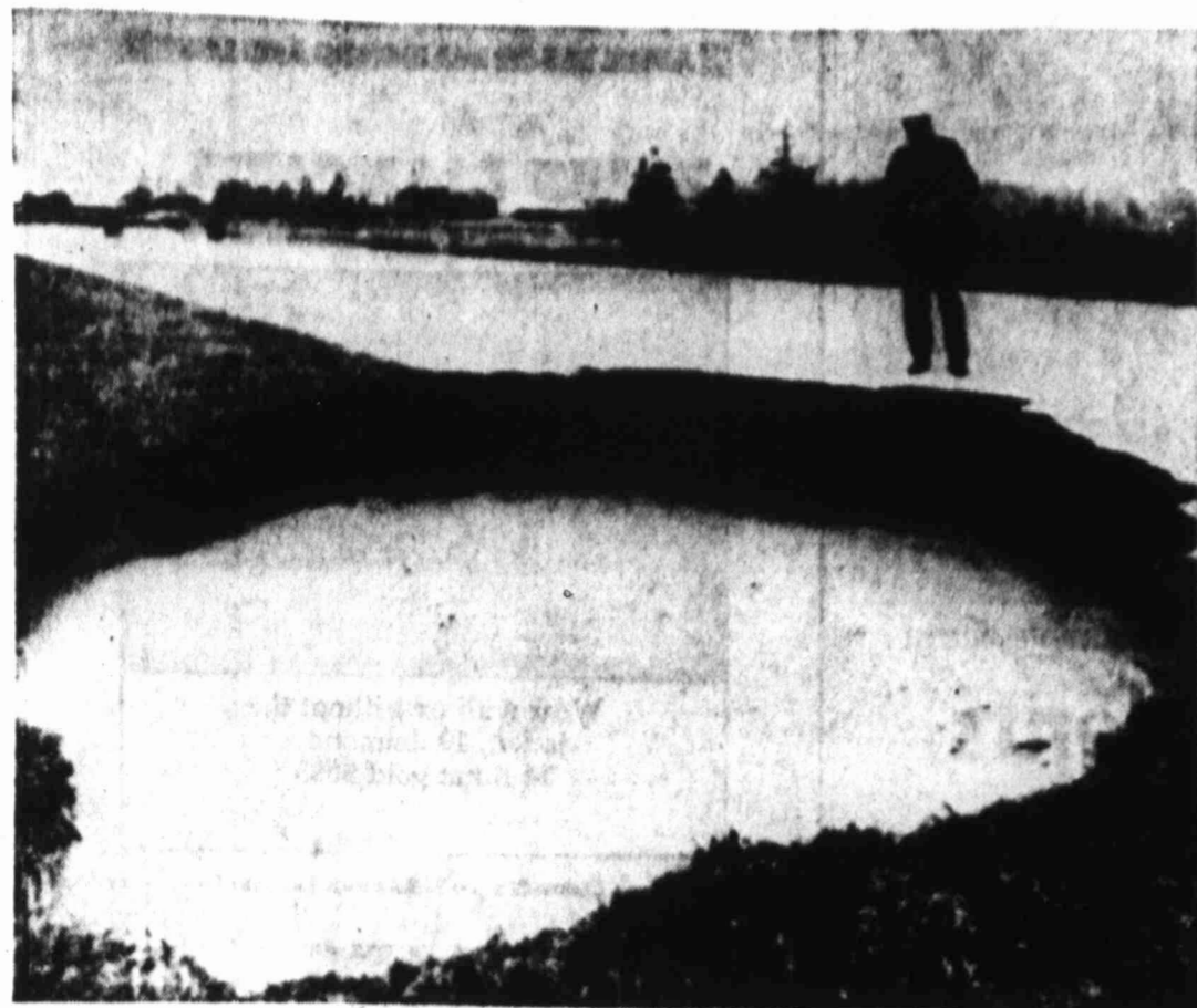
BUBBLING CRATER — A Michigan police Sergeant, William Ogden, stands beside a bubbling crater along highway M72 near Williamsburg, Mich. Several families have been evacuated as geysers and potholes continued to appear. A state official blamed escaping gas from nearby drilling operations for the phenomenon.
