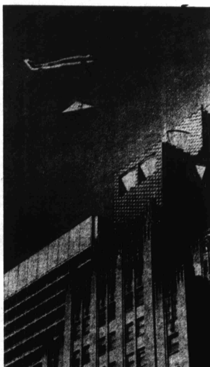
EASY NOW — A helicopter gently lowers a 2,000-pound microwave horn to the telephone building in downtown Oklahoma City. The 10-by-16-foot horn will become part of a microwave telephone relay system to Enid and northwest Oklahoma.
