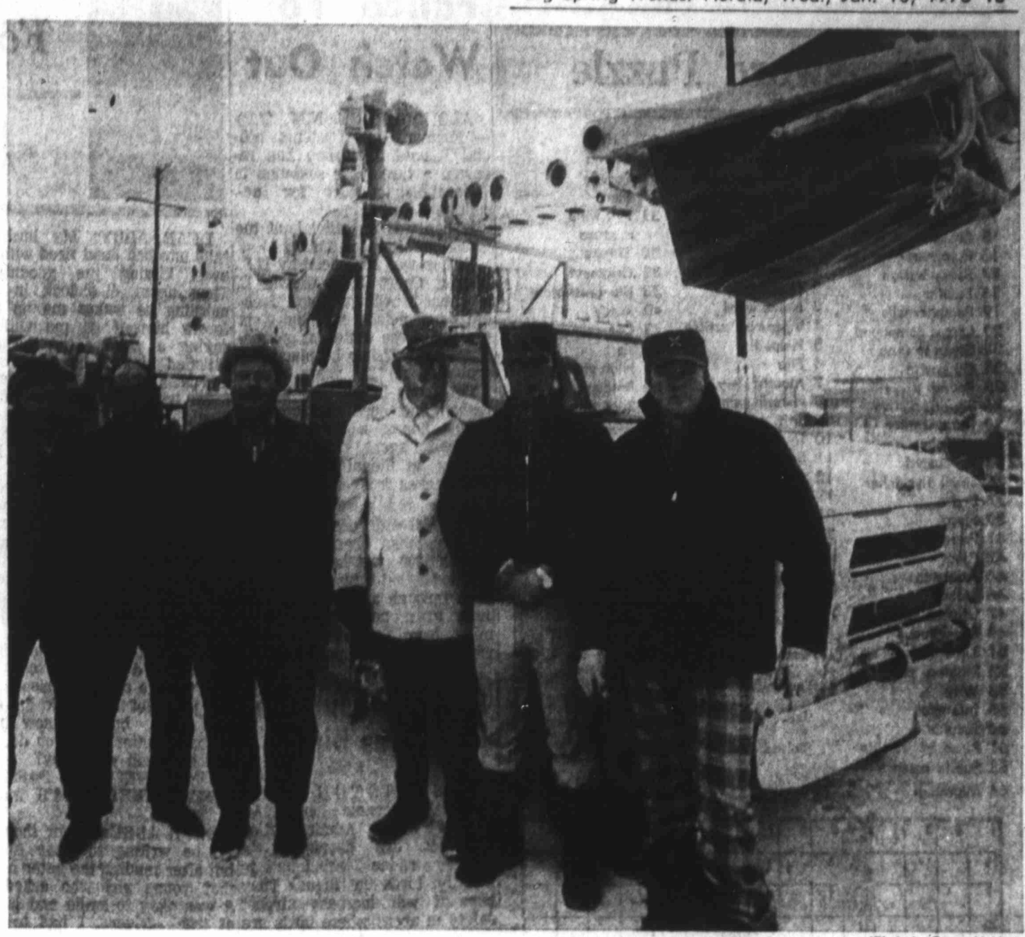
FANNING OUT OVER AREA—Telephone repair crews from Amarillo, Pampa and other points gathered at Southwestern Bell Telephone's service department here this morning before fanning out over the area to repair lines made inoperable by ice storms.
